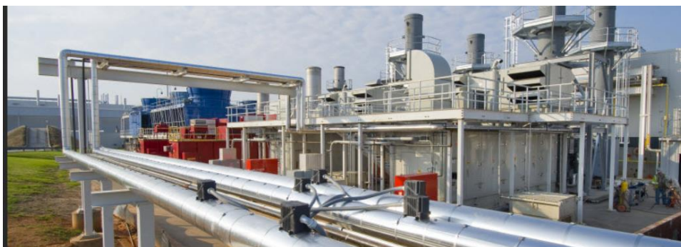
Figure 3. Above-ground pipe installation
