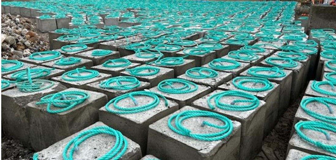
Figure 4: Concrete blocks. Approximately 55 concrete blocks, each weighing 250 kg, are attached to each unit.
