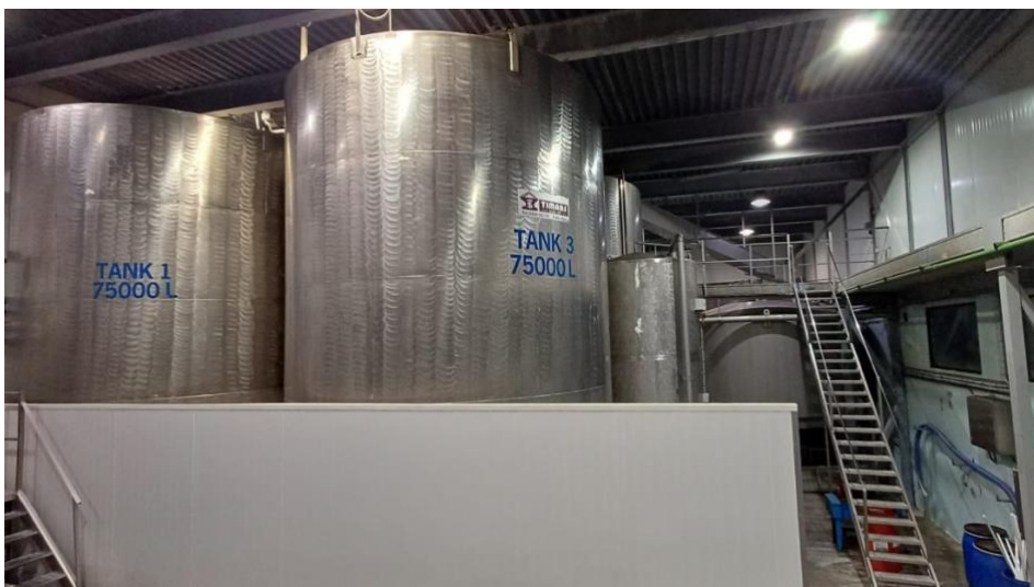
Figure 14: Underutilised infrastructure at the Baltic Sea factory, originally developed for the fishing industry.
